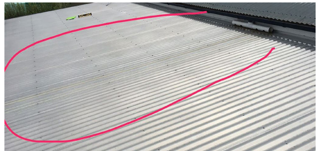
Figure 1. Runoff from the galvanized roof above is causing corrosion to start on this new Zincalume roof 8
