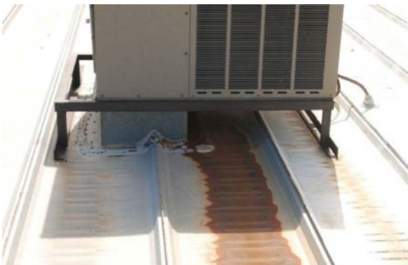
Figure 3. Insufficient corrosion protection on the mounting frame and condensate have damaged this Zincalume roof.
