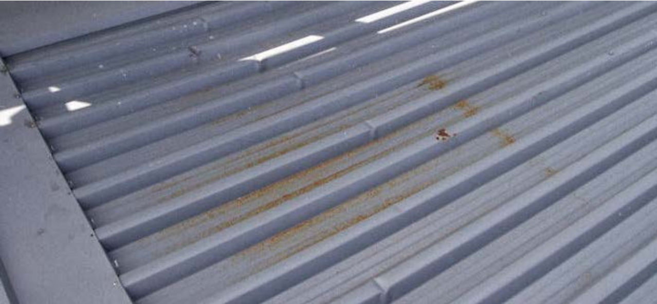
Figure 5. Metal swarf damage due to improper work practices
