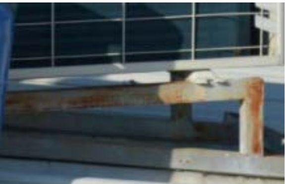
Figure 4. Insufficient corrosion protection on this bracket is beginning to cause roof damage.
