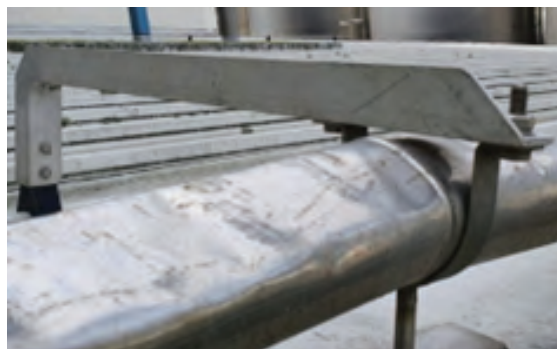
FIGURE 5 CONNECTIONS OF ALUMINIUM TO STAINLESS AFTER 16 YEARS OF DAIRY PLANT ENVIRONMENT
