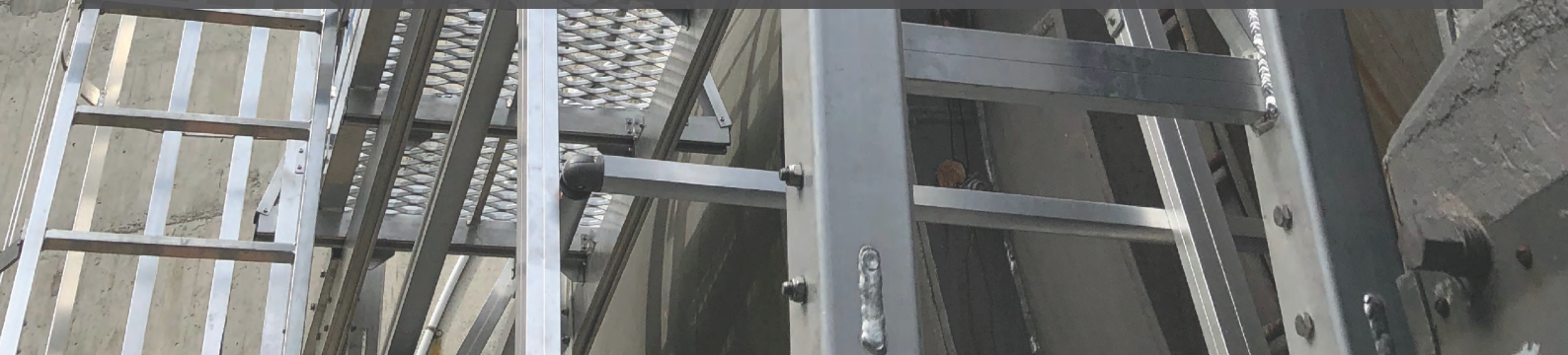
Figure 7 Low Maintenance solution with Aluminium and galvanised components raised above the wet zone
